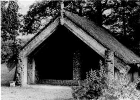
*Figure 5. 1960s Hinemihi following restoration in which a new roof was constructed, the carvings were repainting and the open structure retained.*
